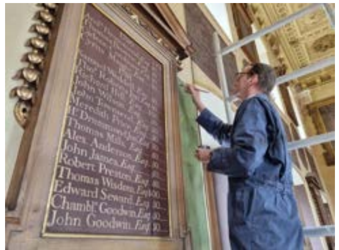
Historic paint specialist Patrick Baty applies colour samples to the walls of the Great Hall ahead of the restoration project.
